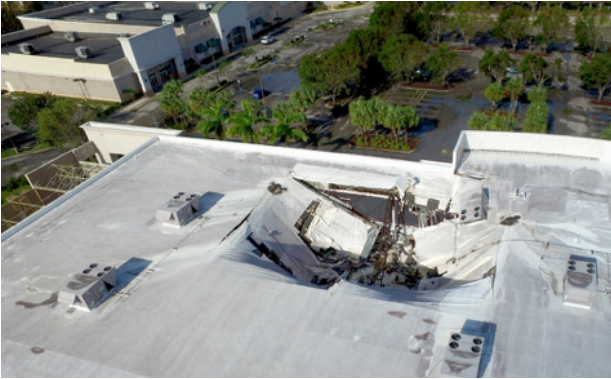
The image above shows damage from a collapsed roof at a warehouse in Florida. The damage was caused from heavy rains resulting from Hurricane Irma. The photo, and many others around the property, was taken via drone.
